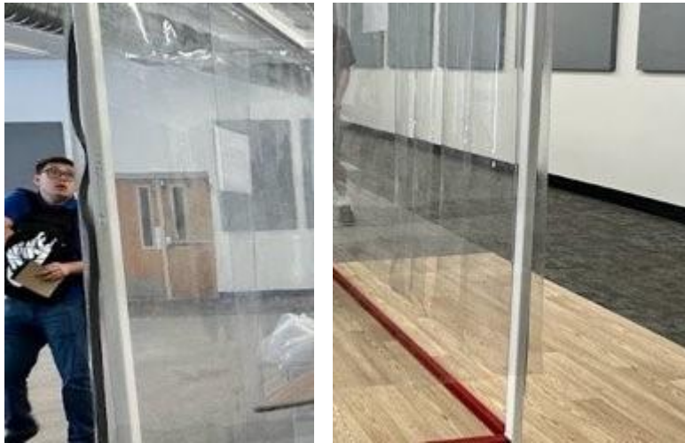
Figures 12-13: A closer look at the effects of time on the current soft wall cleanroom
